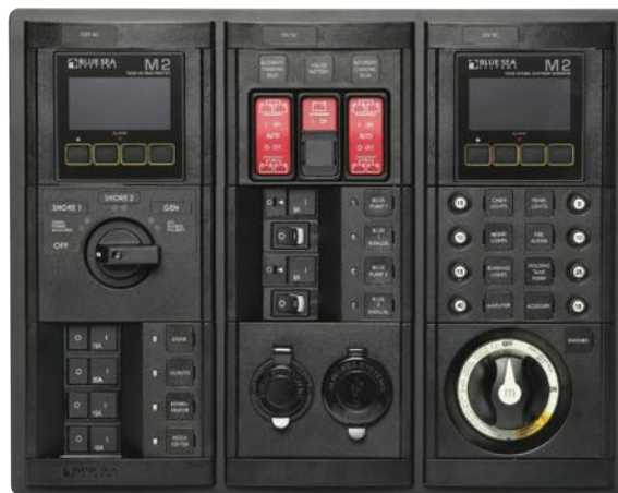
Completed 3 x 3 Panel
